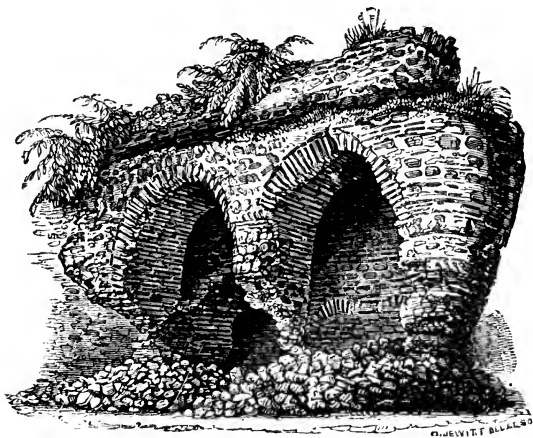
PART OF THE ROMAN WALL AT LEICESTER.
